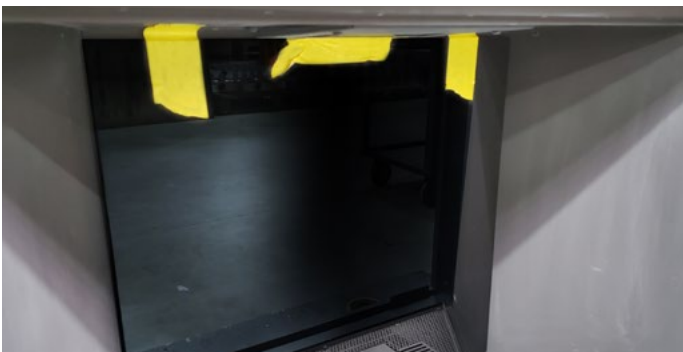
Figure 20.b hold it in place using masking tape
