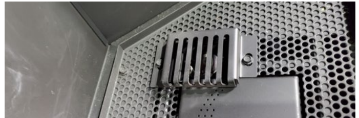
Figure 13. Removal of pilot cover
